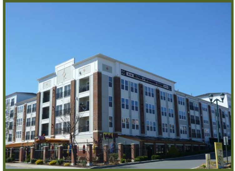
100 Park at Wyomissing Square
