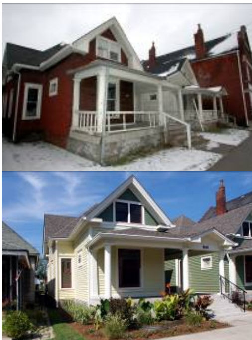
Figure 8 & 9: SEND housing project, before and after renovation Photo: Paul Baumgarten
