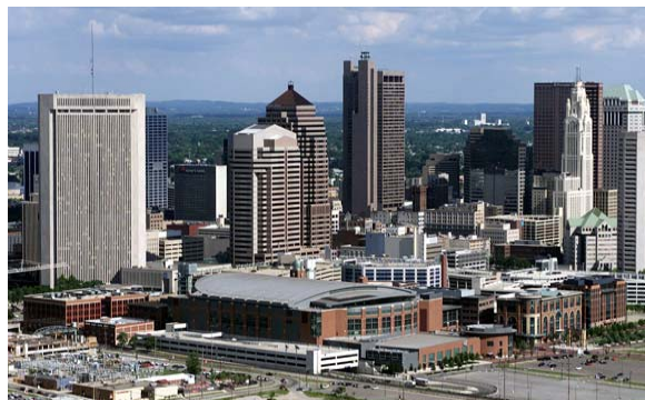
Figure 1: View of the Arena District
