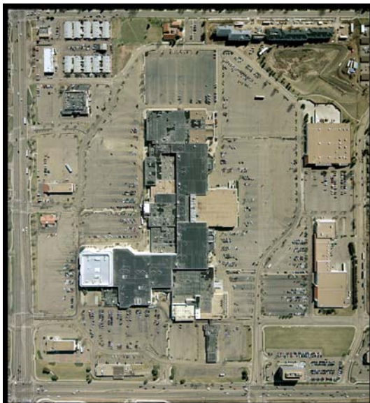
Figure 1: Aerial view of former Villa Italia Mall
