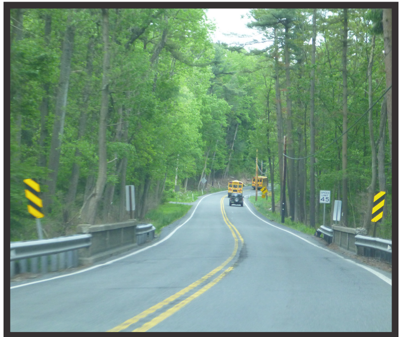
Bridge on Route 625 in Cumru Township over Angelica Creek
